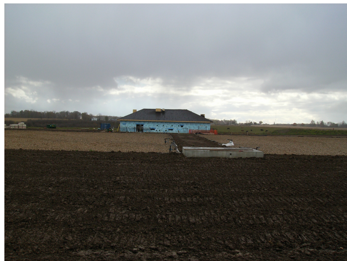
Figure 3. Completed SAGR process with insulating woodchips at grade
