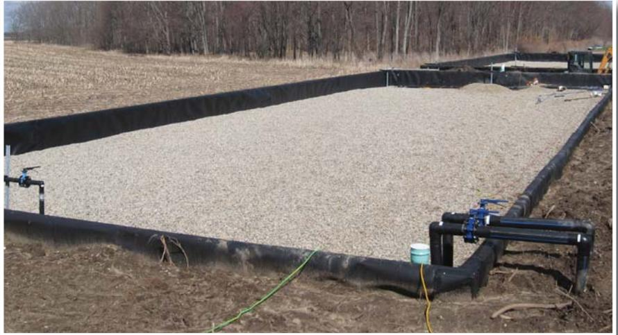
Mentone's SAGR (Submerged Attached Growth Reactor).
